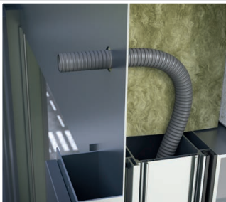
Guide the protective conduit through the facade
